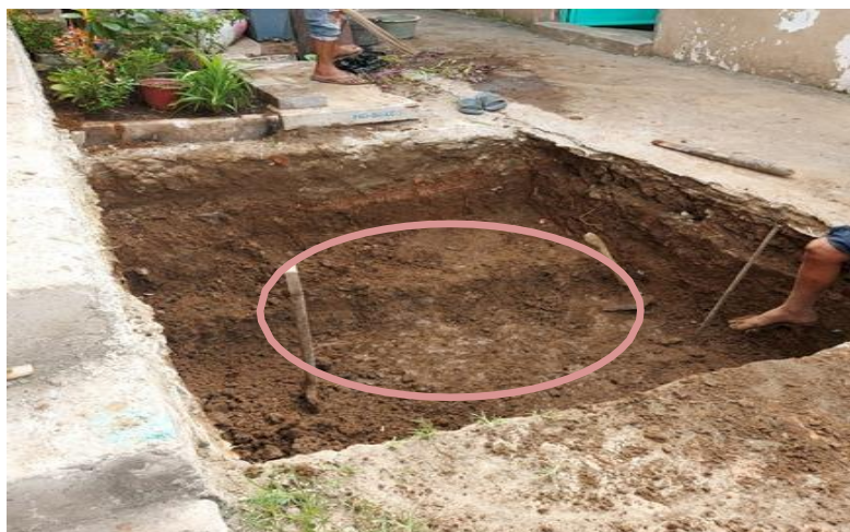
Figure 3. Excavation for making rainwater harvesting
