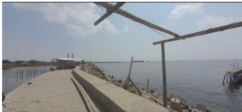
Figure 5. Condition of Marunda Beach
