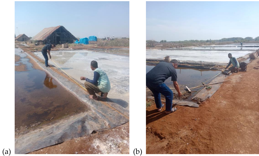
Figure 5. Measurement of the land where the salt tunnel will be built, (a) measurement of the length and width of the crystallization table, (b) measurement of the length and width of the old water tendon.
